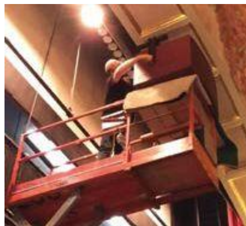
Kent Laabs of Soundworks Systems installs the new balcony speaker cluster.
