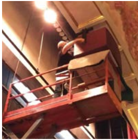
KENT LAABS OF SOUNDWORKS SYSTEMS INSTALLING THE CENTER CLUSTER
